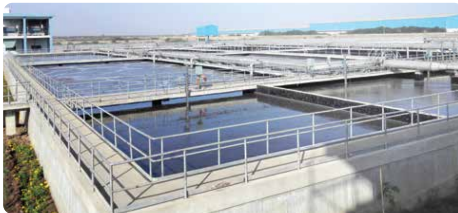
30 MLD Sewage Treatment Plant
