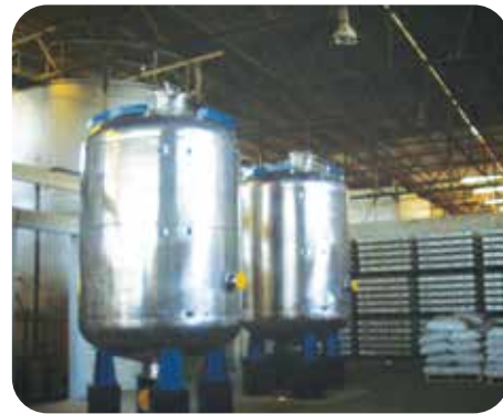
Activated Carbon Filters at Pepsi, Bahrain
