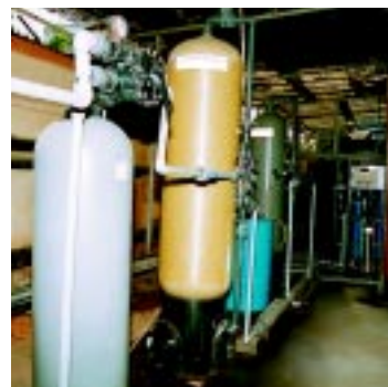
For drinking water, RO system of 0.6 m 3 /h capacity, with full pretreatment consisting of filtration, iron removal, activated carbon, softening and ultra violet sterilisation, at Defence Complex, Hastings, Kolkata.
