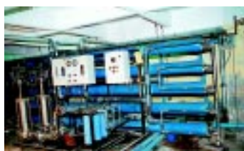
20 m 3 /h reverse osmosis (RO) system for drinking, cooling tower and boiler purposes at CGO Scope Office (20,000 inhabitants) at Lodhi Road, New Delhi. Five year annual maintenance contract.
