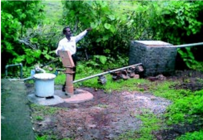
Rooftop rainwater harvesting at Tondsure.
