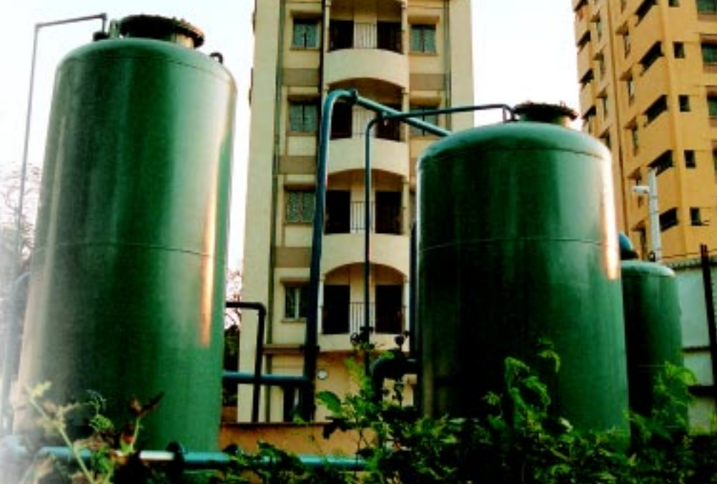
20 m 3 /h reverse osmosis (RO) system for drinking, cooling tower and boiler purposes at CGO Scope Office (20,000 inhabitants) at Lodhi Road, New Delhi. Five year annual maintenance contract.
