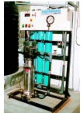
For drinking water, RO system of 0.6 m 3 /h capacity, with full pretreatment consisting of filtration, iron removal, activated carbon, softening and ultra violet sterilisation, at Defence Complex, Hastings, Kolkata.
