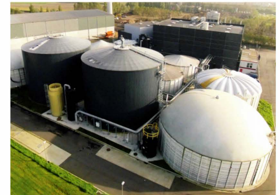
Sludge Digestion - Waste-to-Energy
