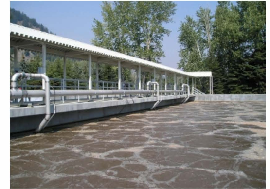
Drinking Water Treatment for Municipality
