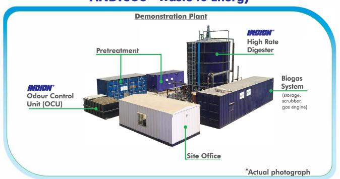
The above plant is designed to treat approximately 1000 kg of organic waste generated by a community kitchen and  $2 - 6 \text{ m}^3$  of sewage sludge per day. It is expected to produce 20 KW/h of electrical power and about 1.35 tonnes per day of organically rich fertiliser.
